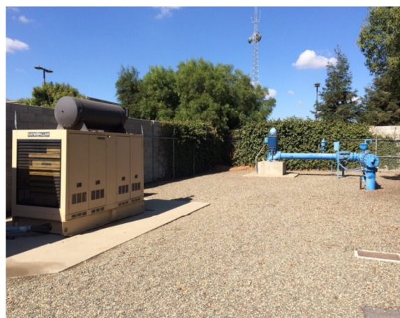
Well Site No. 3A
