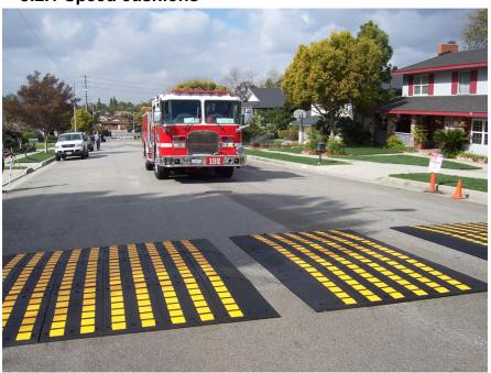
Speed cushions are similar to speed humps or speed tables that include wheel cutouts to allow large vehicles to pass unaffected, while reducing passenger car speeds. They can be offset to allow unimpeded passage by emergency vehicles and transit buses, and are typically used on key emergency response routes. Speed cushions extend across one direction of travel from the centerline, with a gap to allow wide wheelbase vehicles to avoid going over the hump.
