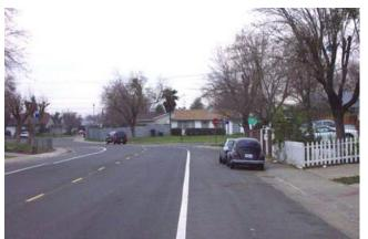
Edgeline striping is used to create narrow travel lanes which give the impression of a narrow street, which may help reduce overall speeds. Striping can placed near the curb, center of roadway, or midblock to create the appearance of a constricted roadway. Edgeline striping is effective on long, wide residential streets with speeding traffic, although it may result in loss of street parking.
